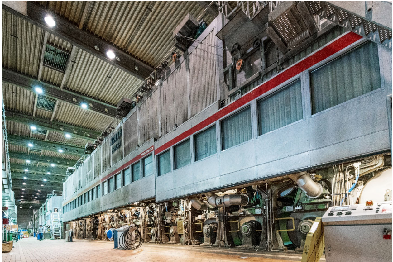
Figure: Paper machine 5 after rebuild phase 1, Oberkirch, Germany
