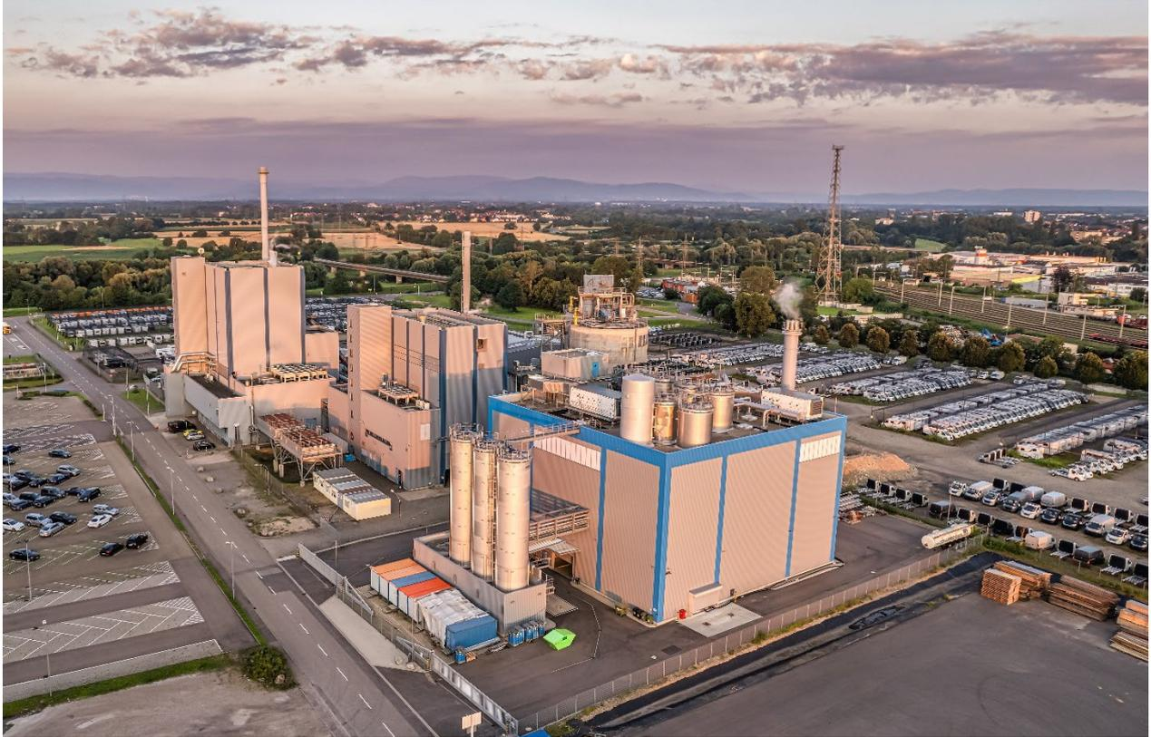
*Figure: The two biomass combined heat and power plants supply process steam to the paper production processes at the Koehler Paper site in Kehl. / Image rights: Koehler Group*
