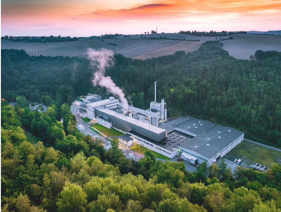
Figure 2: The Koehler Paper site in Greiz. Source: Koehler Group
